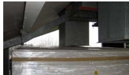
Precision Installation of the new Chillers
