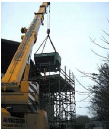
Removal of the existing chillers, via the 7 meter load platform
