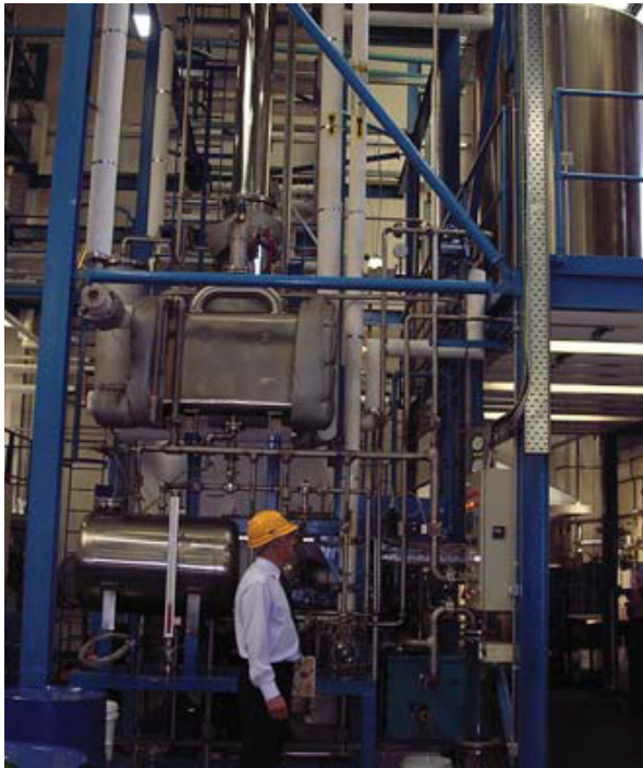
Chris Dimmick inspects the plant
