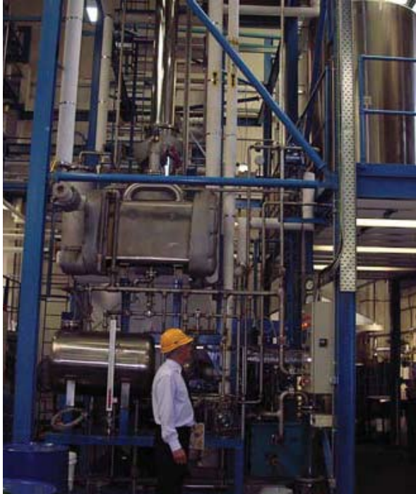
Chris Dimmick inspects the plant
